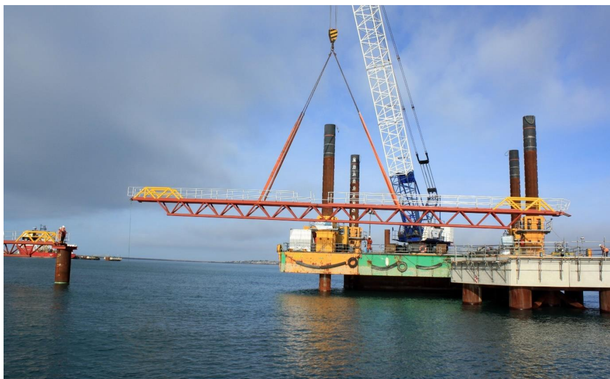
Picture: Final walkway being moved into position
